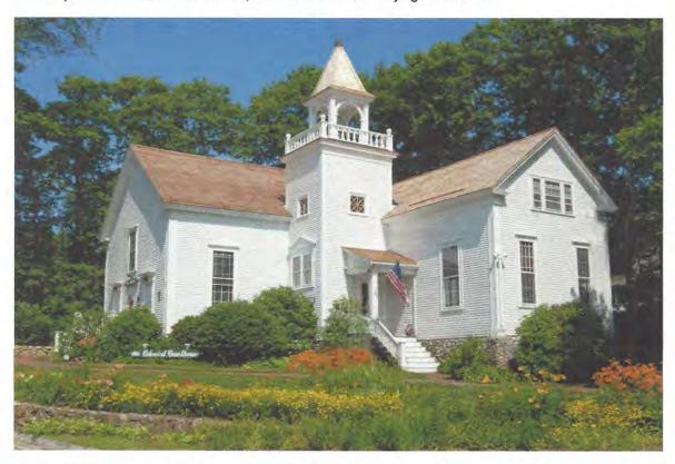
The railing that surrounds the belfry of the 1905 bell tower was reconstructed as part of the 2019 restoration project. At the time of this project, Tales of Cape Cod was unable to locate any architectural drawings, measurements, or pieces of the original railing. The design for this reconstruction was taken from a photograph (circa 1905).
