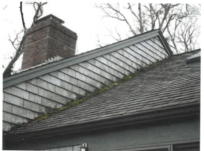
Roof cleaning and shingle repair
