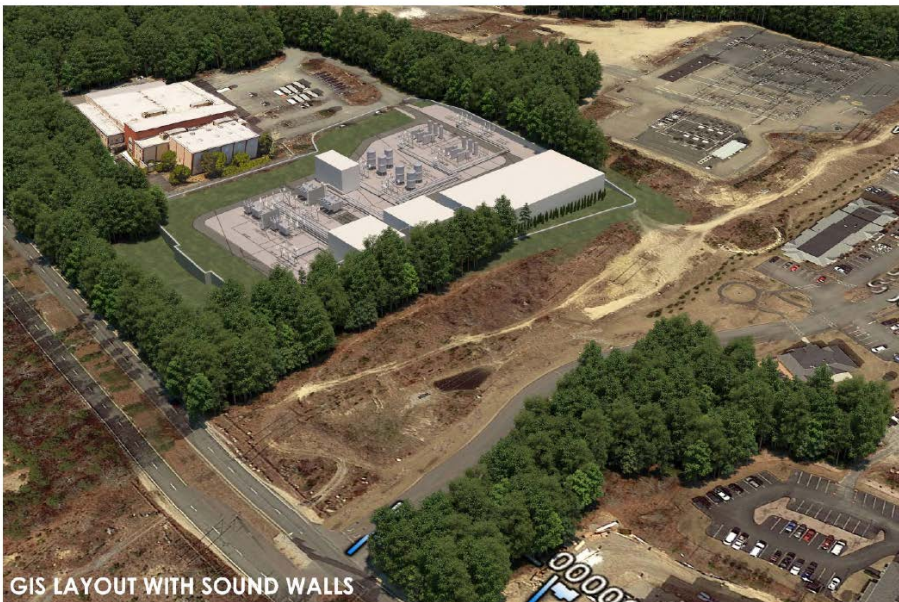
Figure 7. GIS Layout with Sound Walls
